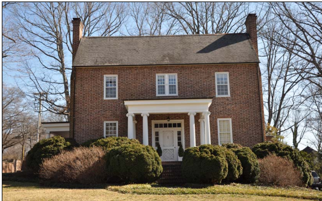
Figure 9: This two-story Flemish-bond brick house is an excellent example of an early nineteenth-century brick house in Henry County. Known as Greenwood, (120-0002) , it was built for Col. Joseph Martin in 1810 and moved from Axton to Martinsville on Mulberry Road around 1940. Martinsville was named for his father, General Joseph Martin.
